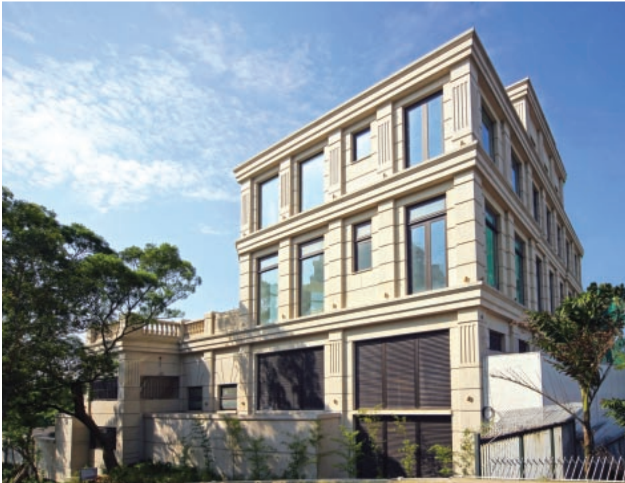
▲ Construction of the residential development at 78 Mount Kellett Road 興建加列山道78號住宅發展項目
