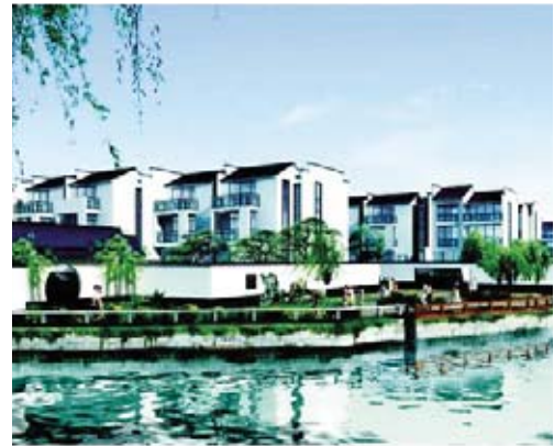
Semi-detached townhouses nestled amongst a natural environment and spectacular scenery 半獨立式住宅處身優美的大自然風景區
