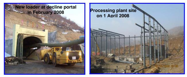
Construction of the processing plant re-commenced in March 2008 with both the plant and tailings dam contractors mobilising to site and commencing steel erection and earthworks. The plant is being built with Chinese equipment and is a standard Chinese design carbon-in-leach plant.
