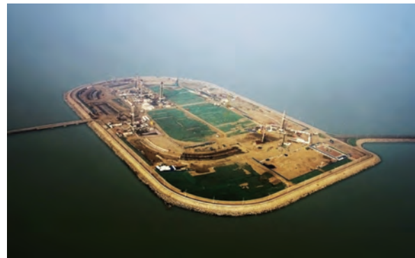
No. 1 Artificial Island Project of Jidong Nanpu Oilfield
