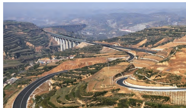
BOT project of Yicheng-Houma Expressway
