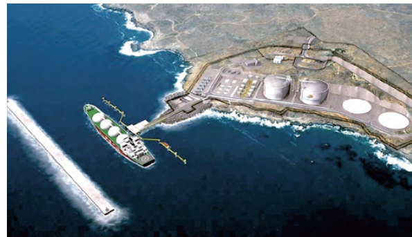
LPG Dock Breakwater Project in Mexico
