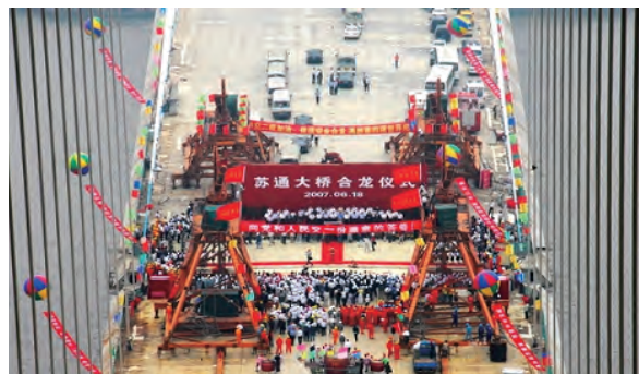
Sutong Bridge was joined in June 2007
