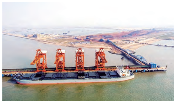
Phase I of Caofeidian Ore Terminal Project
