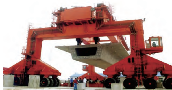
900T rubber-tyred crane for lifting railway girder
