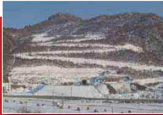
White Mountain decline portal area in January 2008
