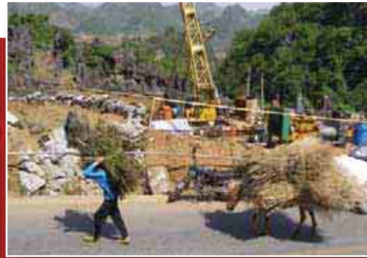
Drilling at Jinluo Joint Venture
