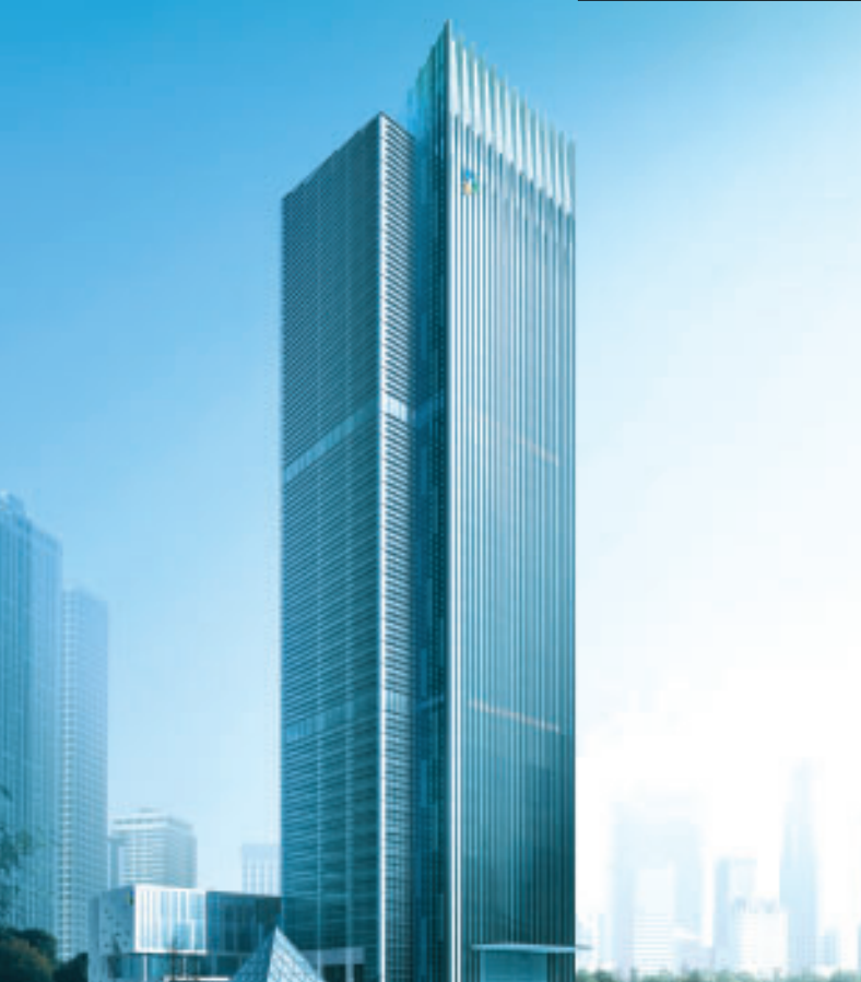
Nantong International Trade Center 南通國際貿易中心 Grade-A office complex in Nantong City 南通市甲級商業大廈
