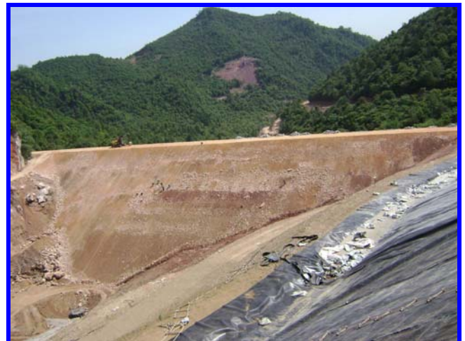
Tailings dam embankment completed
