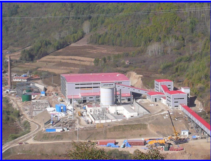
Overview of processing facility
