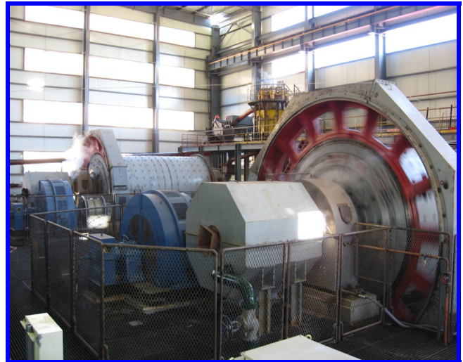
Commissioning of ball mills
