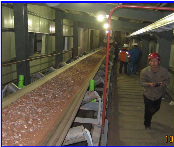
Commissioning of ore conveyor
