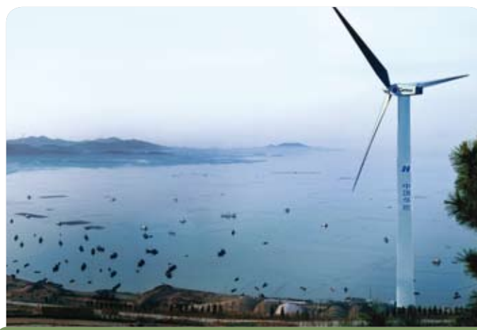
Changdao wind farm in Yantai City, China
