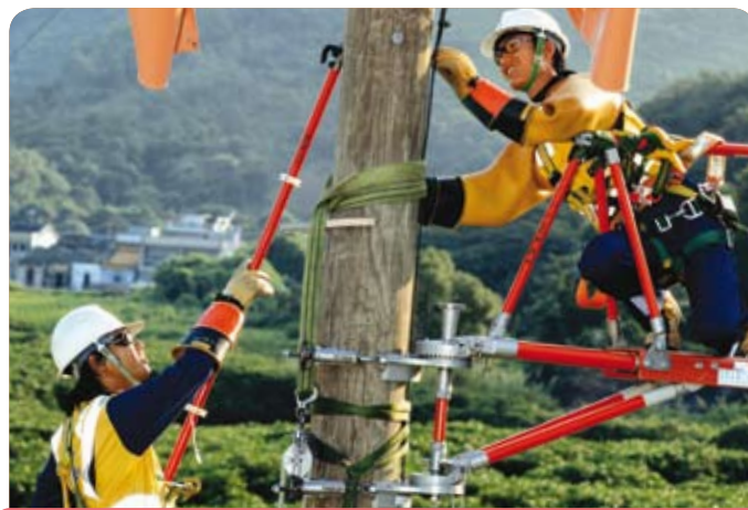
CLP requires employees to be fully equipped with safety harness
