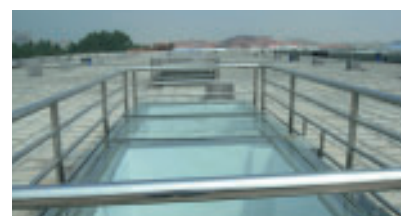
Skylights in the roof to illuminate the building using sunlight. 屋頂上利用太陽光為樓宇照明的光源。
