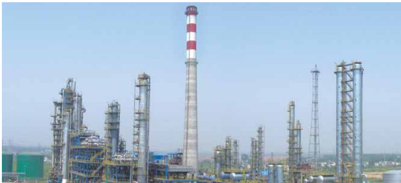
The chemical refinery plant in Yangzhou, Jiangsu province provides new impetus to our chemical division 位於江蘇省揚州之煉化廠為化工部門提供新的增長動力
