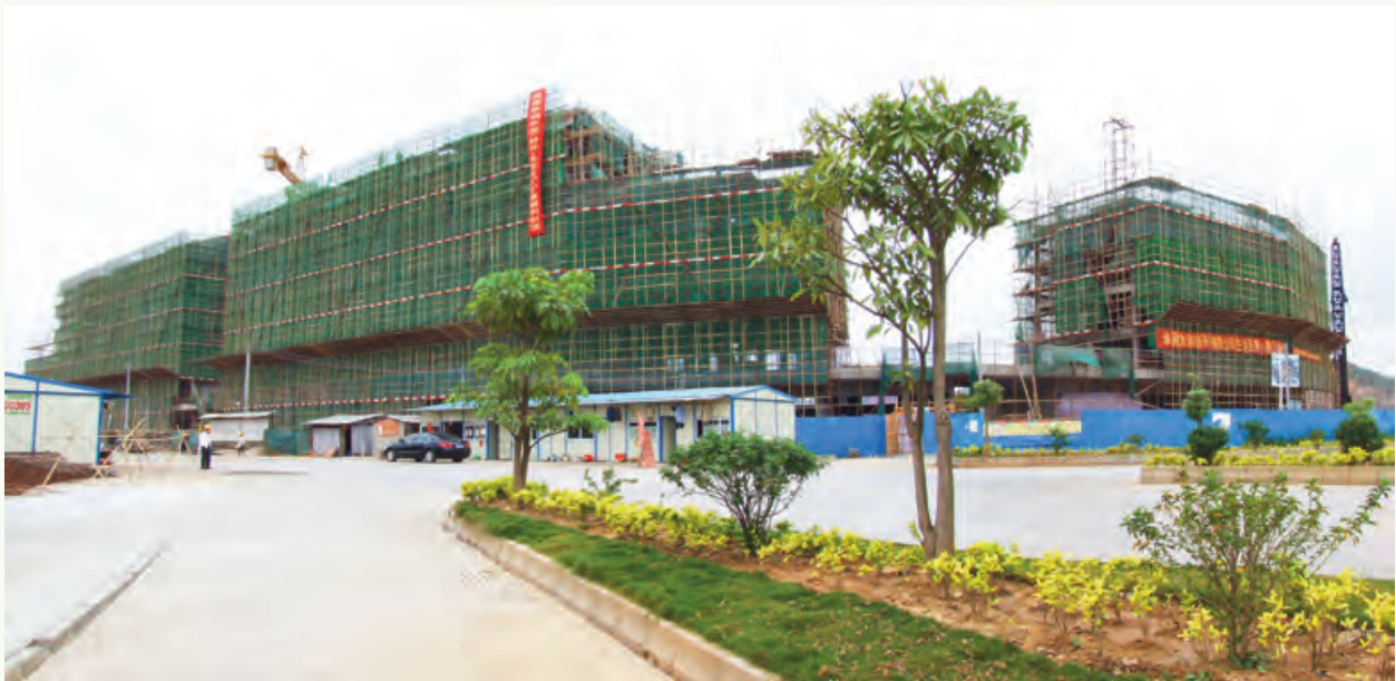
於廣東封開在建中的員工宿舍 Employees' dormitory under construction in Fengkai, Guangdong
