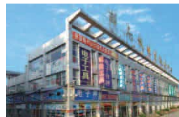
Phase I Electronics and Accessories Trade Center 一期電子原材料交易中心
