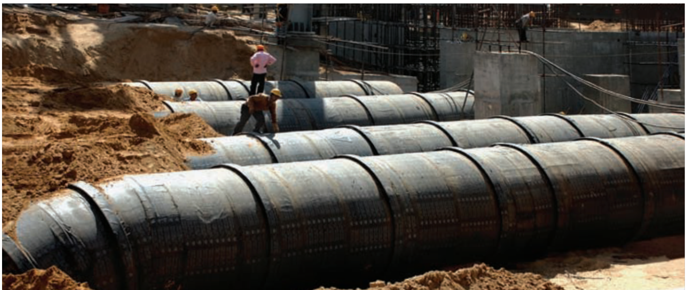
建築工人於哈格爾Mahatma Gandhi熱電廠安放冷卻水管
