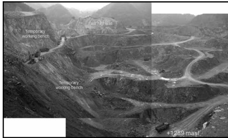
Figure 11.7 Current Pit Status - East
