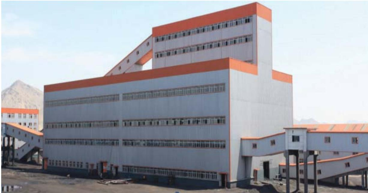
The coal processing plant at Urad Zhongqi uses a dense-medium separation process. The dense-medium separation process has a higher set up cost than the dry separation process and requires a large amount of water at the outset of the operation, but is capable of a more effective separation compared to the dry separation technology. The following flow chart illustrates the process flow of the dense-medium separation process:
