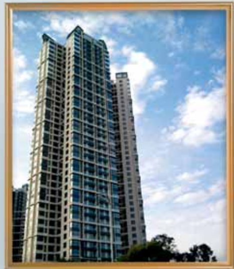
Shanghai International Financial Center (SIFC) Tower 2008-2010 Architect: Skidmore, OWINGS & Merrill LLP Client: Shanghai International Financial Center
