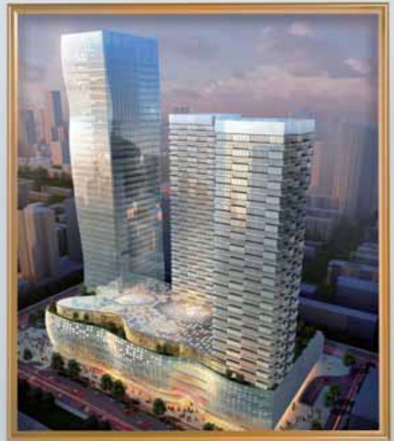
Shanghai International Financial Center (SIFC) Tower 2008-2010 Architect: Skidmore, OWINGS & Merrill LLP Client: Shanghai International Financial Center
