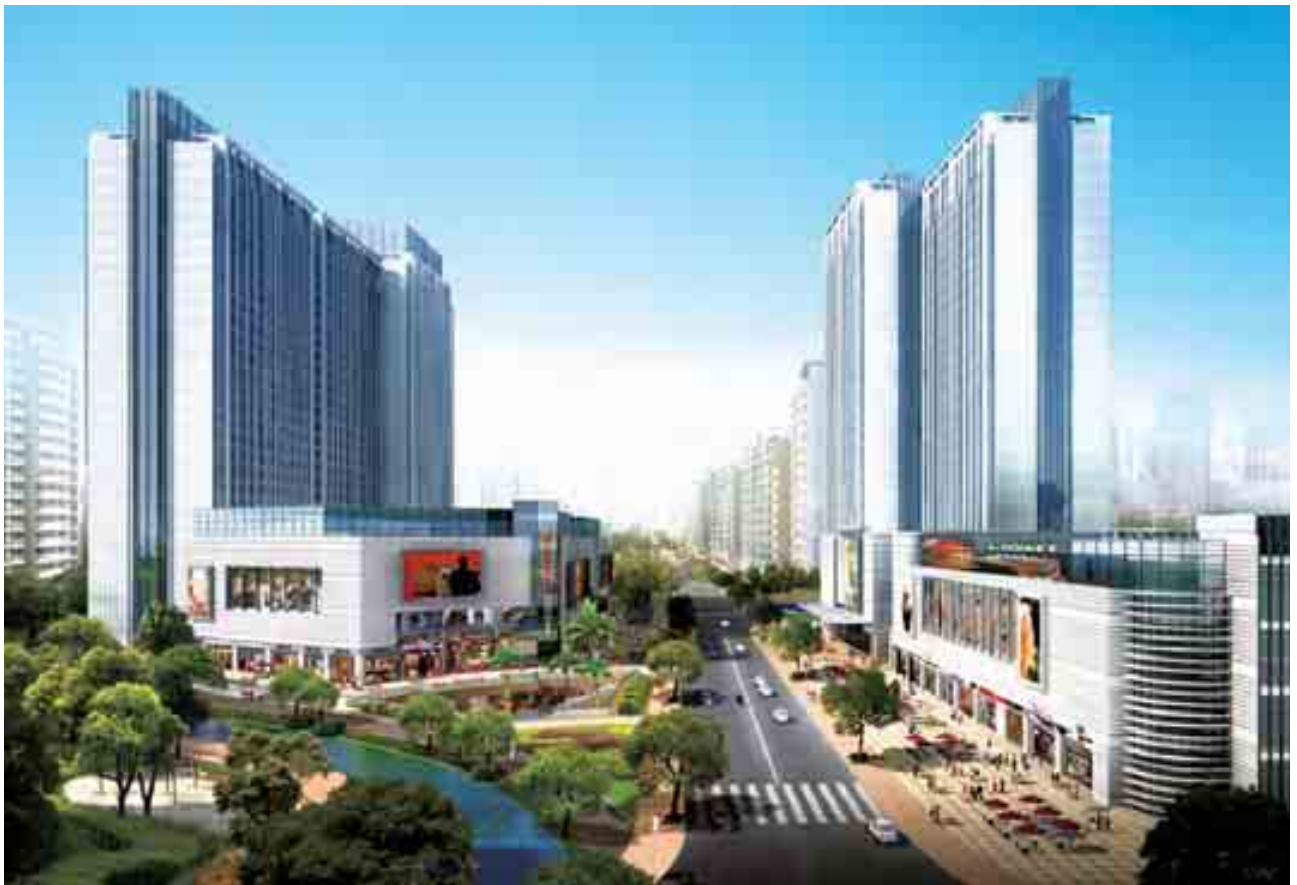
Guangzhou Jiahe Commercial City 廣州嘉和商業城
