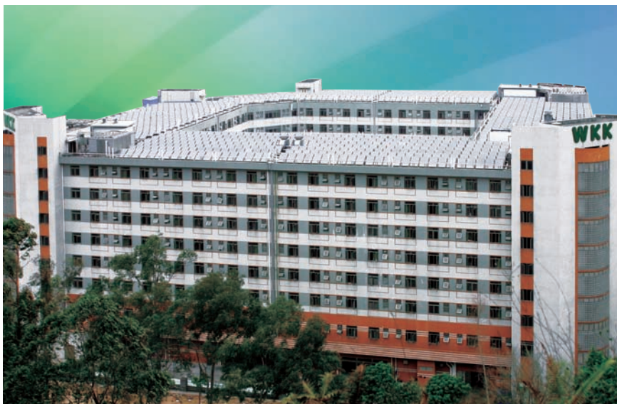
Worker dormitory 工人宿舍
