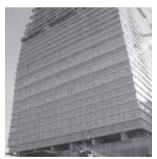
A semi-unitized curtain wall is a type of curtain wall which has the combined features of stick curtain wall and unitized curtain wall. All components of semi-unitized curtain wall except main keels are fabricated and assembled into unitized panels at our production facilities, and then delivered to construction sites to be fixed on main keels for installation.
