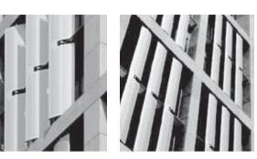
A shading system is used to shield a building from excess sunlight. It helps to improve the energy efficiency of a building by reducing the amount of air conditioning required in the building. We have applied intelligent control technology to some of our shading systems, which can automatically adjust its position in response to the sun's path.
