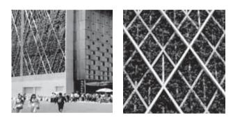
Ecologically friendly curtain wall is a type of ecologically friendly outer building structure that is covered by a botanical layer with a bioclimatic buffering layer. Ecologically friendly curtain walls are designed to achieve resource conservation and reduce pollution.
