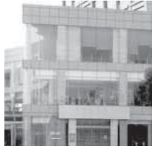
A full-glass curtain wall is another type of non-frame curtain wall where glass panels are connected with each other and eventually connected to the main building through peripheral supporting structures.
