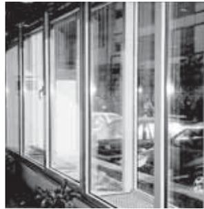
A double-skin energy-saving curtain wall is an outer building structure consisting of an outer curtain wall and an inner curtain wall. It is also known as a dynamic ventilation curtain wall, hot-channel curtain wall and respiration curtain wall. Compared with conventional curtain walls, double-skin curtain walls can effectively improve the thermal insulation of the outer building structure, indoor ventilation, sound insulation and daylighting.
