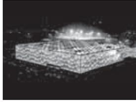
Membrane structure curtain wall is a type of curtain wall that uses high-performance ETFE membrane as its surface material, including ETFE stretching membrane and ETFE aired membrane. The ETFE membrane has many desirable physical features such as high transparency, light weight, high resistance to aging and long life.
