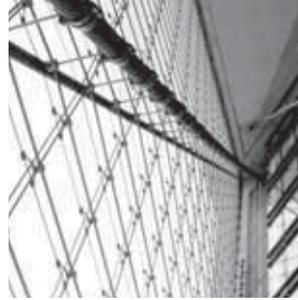
A point-fixing curtain wall is one type of non-frame curtain wall that consists of glass panels, point-fixing components on such panels and their supporting structures.
