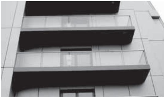
A balustrade/breast board system consists of components which are applied to certain parts of the building, serving the functions of safeguarding and decoration. As an independent system, it is usually applied along the edge of the accessible roof, indoor floor edge and balcony.
