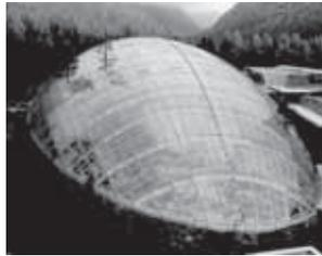
A skylight, which consists of transparent panels and its supporting system, is a roof system that has a horizontal angle of less than 75 degrees. It provides natural lighting for the building and serves other related functions. The transparent panels are usually made of glass, polycarbonate sheet and transparent membrane materials.
