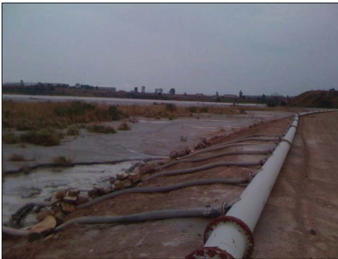
Figure 37: Spigot System Deposition on the eastern flank of the dam
