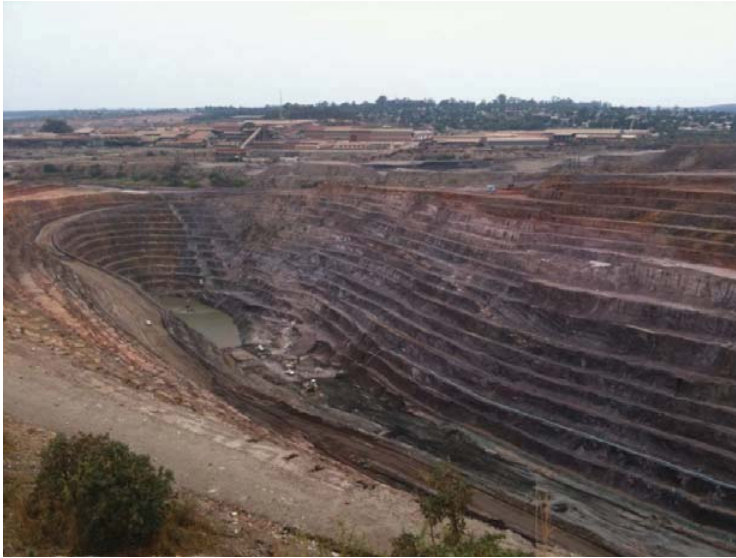
Figure 19: T-17 Open Pit
