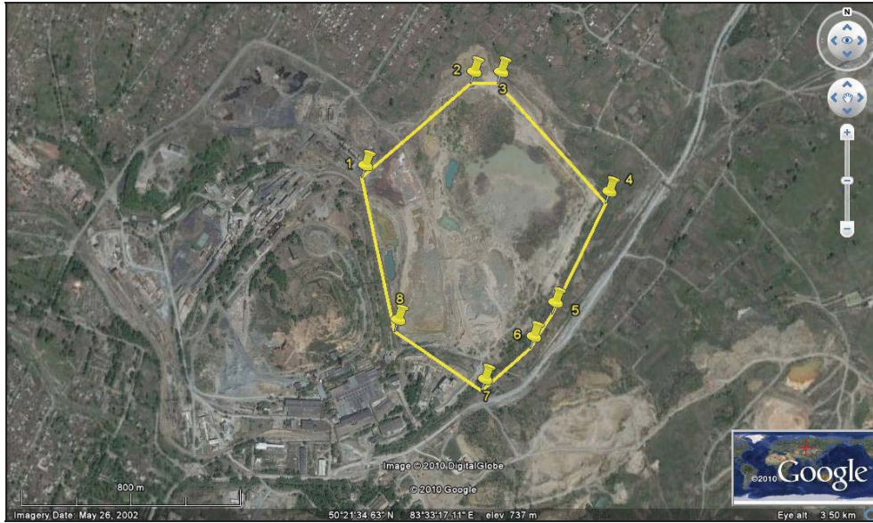
Figure 11.1: Outline of Staroye Tailings Dam
