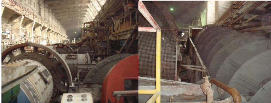
Photo 5.3: Concentrator Building No.3 and Spiral Classifier
