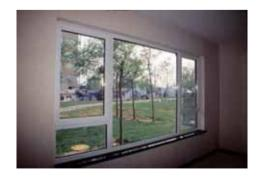
Energy-saving aluminum alloy doors and windows are made of thermal insulation aluminum alloy extrusions and energy-saving glass, all of which can be recycled.
