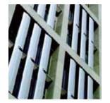
A shading system is used to shield a building from excess sunlight. It helps to improve the energy efficiency of a building by reducing the amount of air conditioning required in the building. We have applied intelligent control technology to some of our shading systems, which can automatically adjust its position in response to the sun's path.
