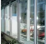
A double-skin energy-saving curtain wall is an outer building structure consisting of an outer curtain wall and an inner curtain wall. It is also known as a dynamic ventilation curtain wall, hot-channel curtain wall and respiration curtain wall. Compared with conventional curtain walls, double-skin curtain walls can effectively improve the thermal insulation of the outer building structure, indoor ventilation, sound insulation and daylighting.
