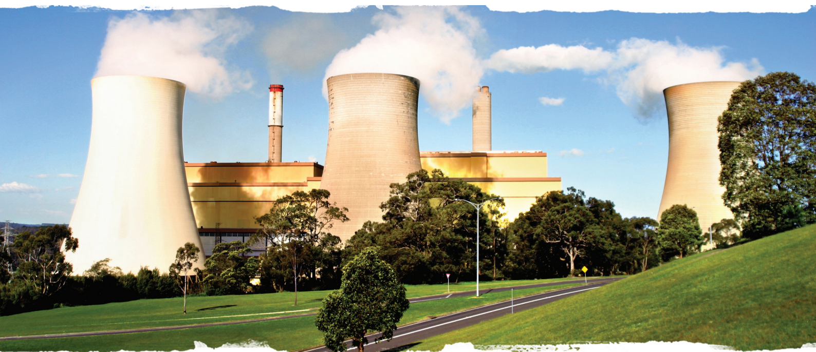
Yallourn Power Station
