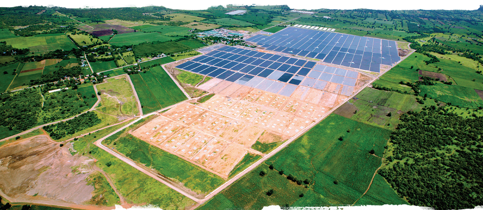
Lopburi solar project
