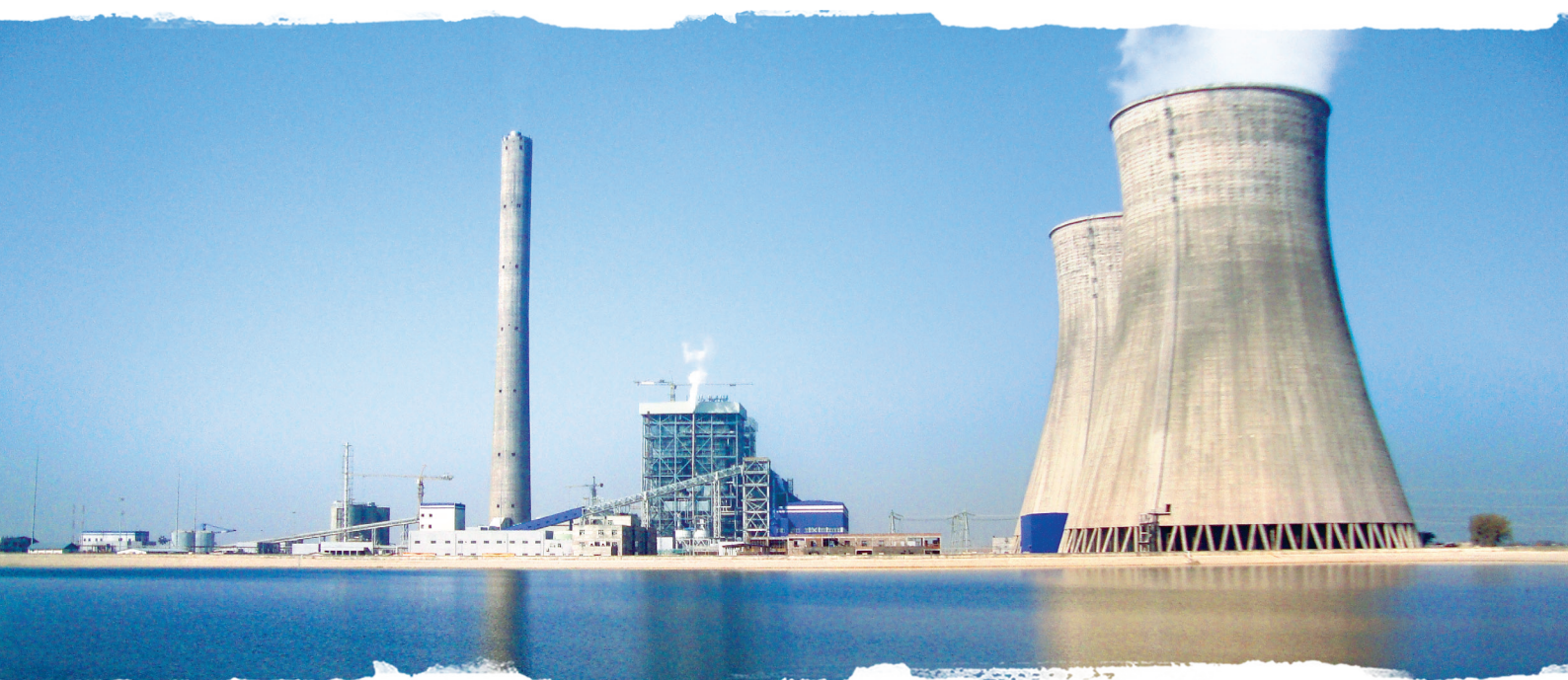
Jhajjar Power Station
