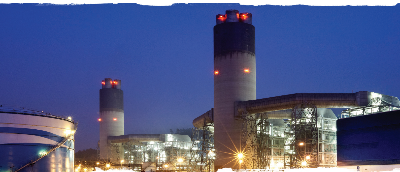
Black Point Power Station
