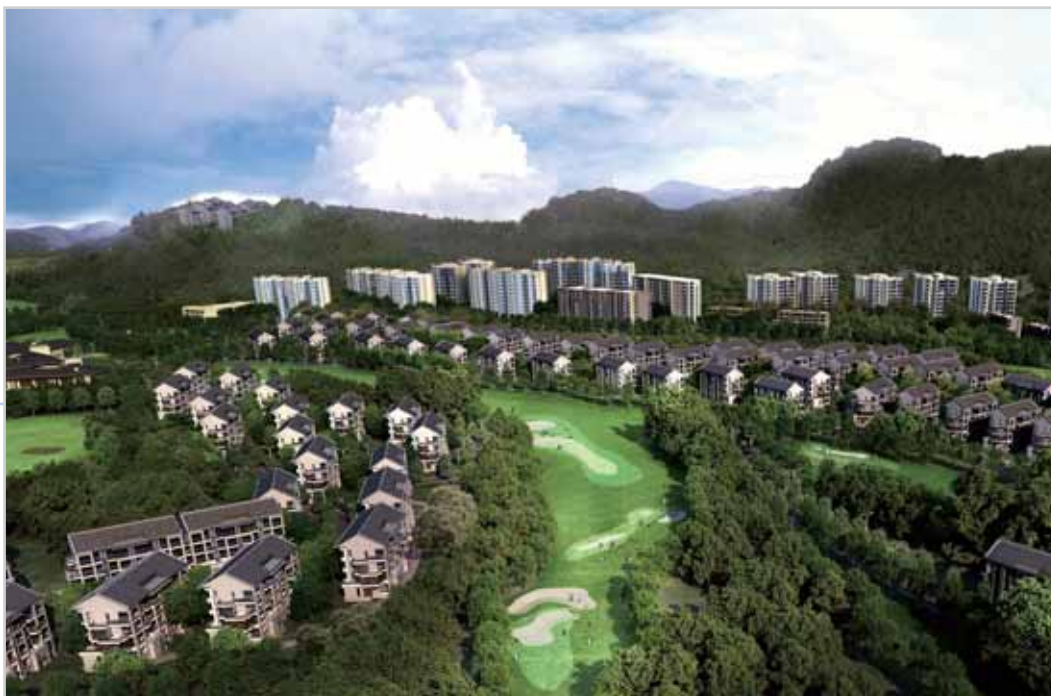
福州天安登雲山莊(鳥瞰效果圖) Perspective of Fuzhou Tian An Dengyun Resort (Aerial View)
