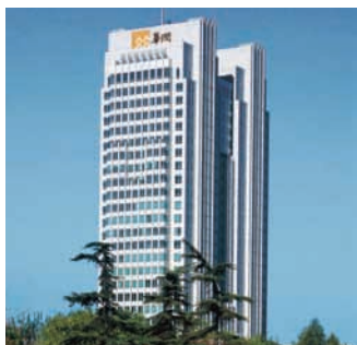
北京華潤大廈 Beijing CR Building
