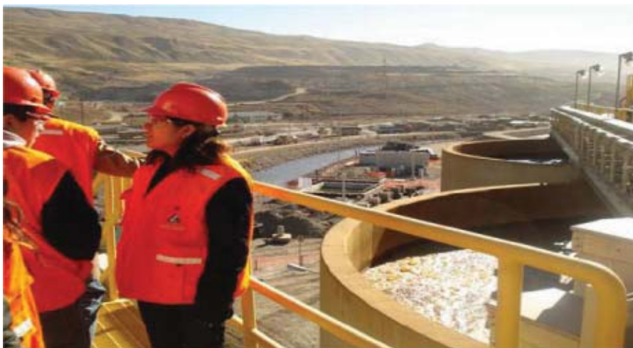
Figure 13.5. The Kingsmill Tunnel Water Treatment Plant facility (Appears to be functioning well with quality construction to treat historic mine drainage in the Toromocho peak area and supply process water for the new mining project)
