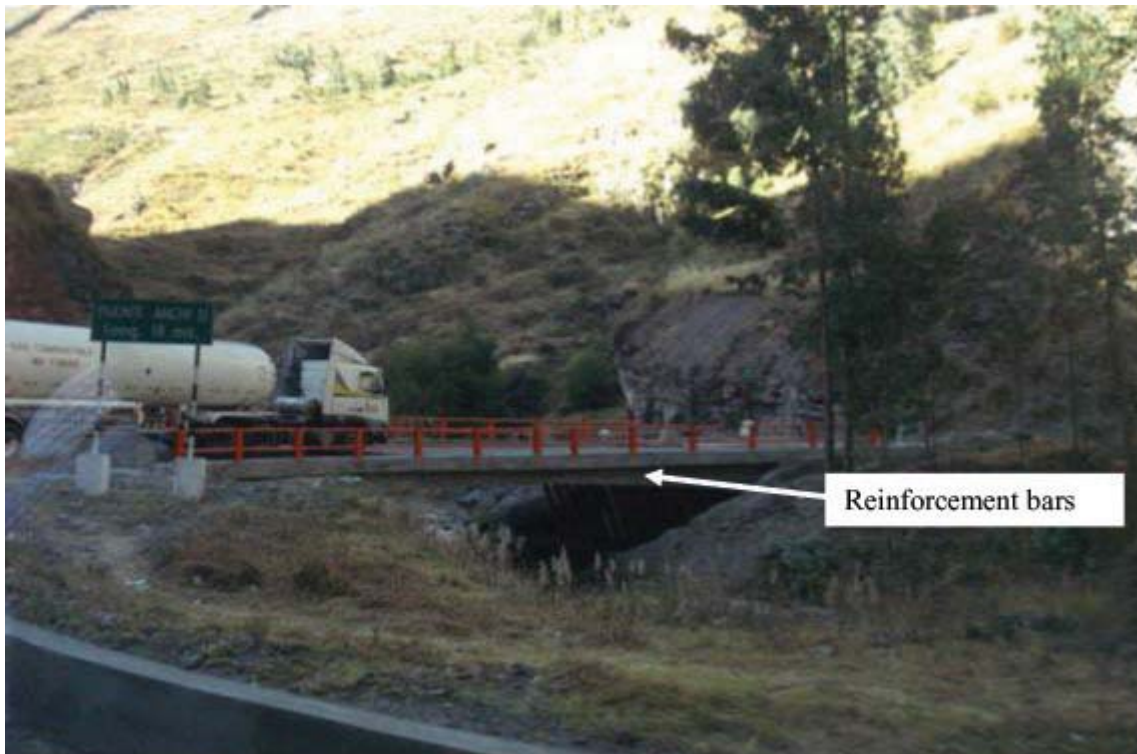
Figure 13.8. Conditions on the Central Highway from Lima (Include new bridge improvements, with the red reinforcement bars under the bridge platform (barely visible below the platform at right) supplied by MCP to handle their major shipments of equipment and supplies)
