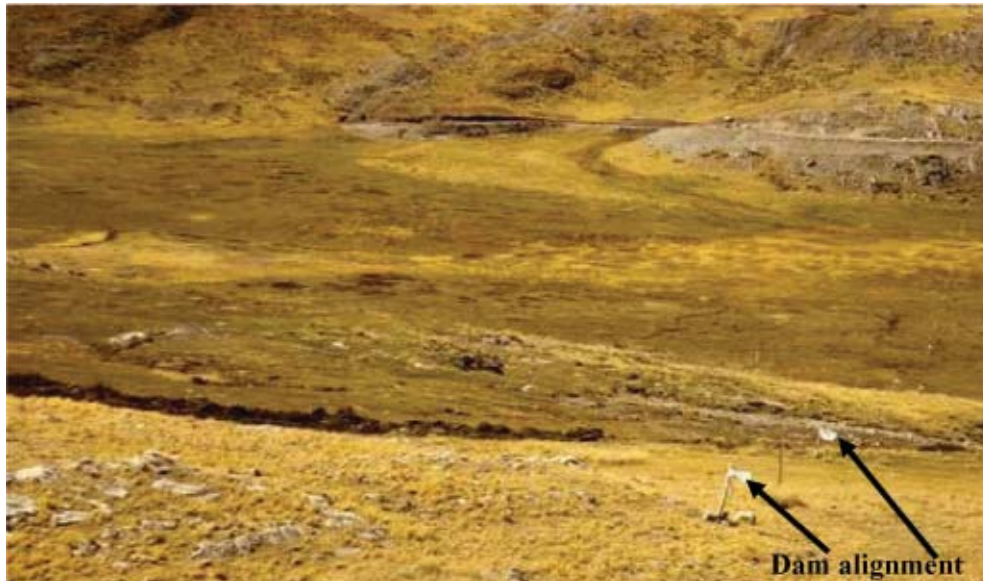
Figure 13.4. Wet, marshy soils (“bofedal”) are being removed from the margin of the tailings dam construction area in the Tunshuruco valley (Alignment of the dam is shown in the flags at the right)
