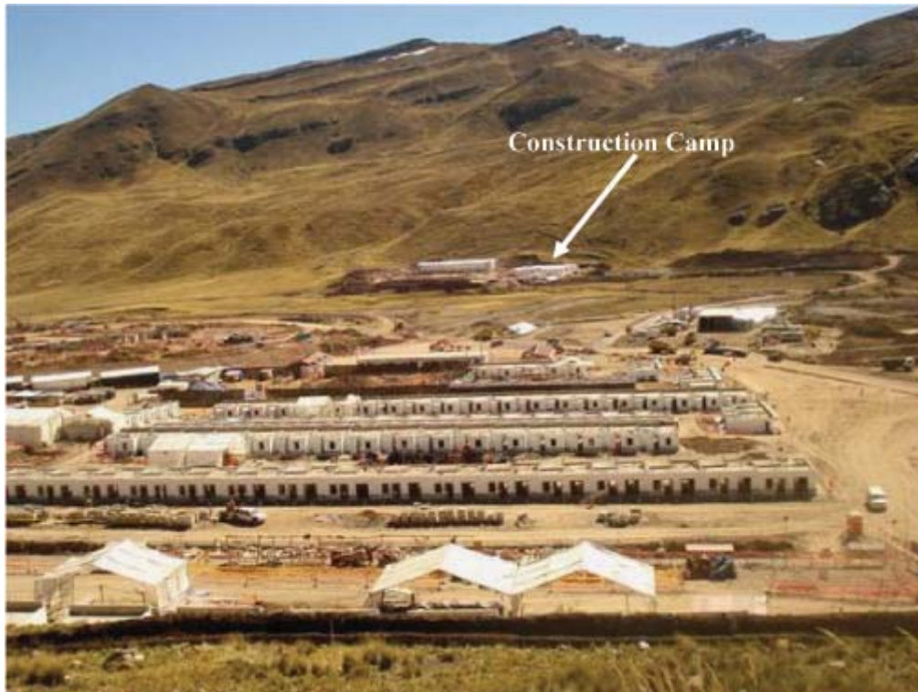
Figure 13.7. The new town at Carhuacoto (Well under construction in the foreground with a construction camp being developed in the background against the ridge)
