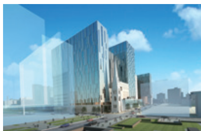
蒙特婁University of Montreal Hospital Centre
