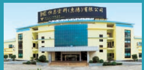
位於廣東惠州的塗料廠房 The coatings plant in Huizhou, Guangdong
