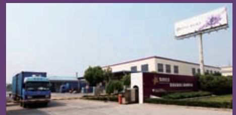
位於上海青浦的塗料廠房 The coatings plant in Qingpu, Shanghai
