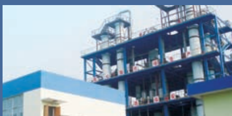
位於廣東江門的溶劑廠房 The solvents plant in Jiangmen, Guangdong
