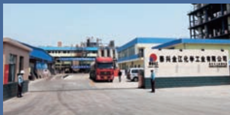
位於江蘇泰興的溶劑廠房 The solvents plant in Taixing, Jiangsu
