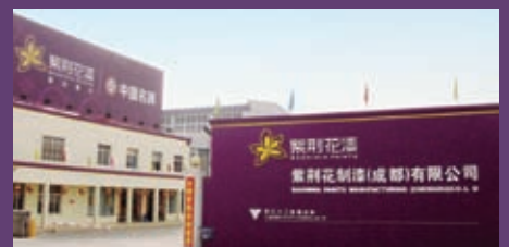
位於四川成都的塗料廠房 The coatings plant in Chengdu, Sichuan
