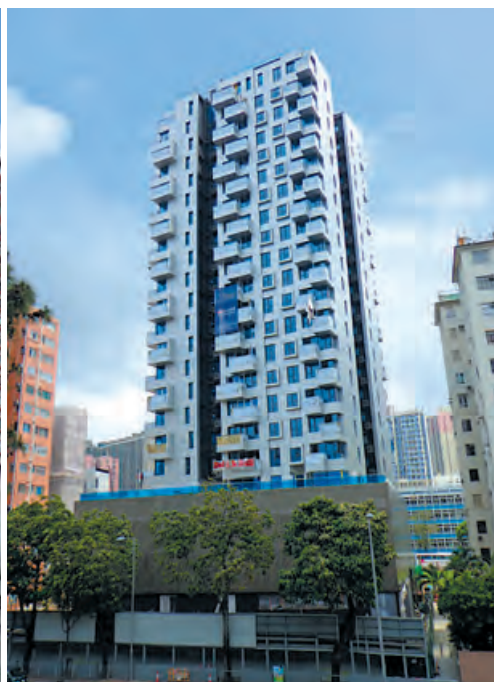
Proposed residential redevelopment at Nos. 146 & 148 Argyle Street, Kowloon 九龍亞皆老街146及148號的建議住宅重建項目
