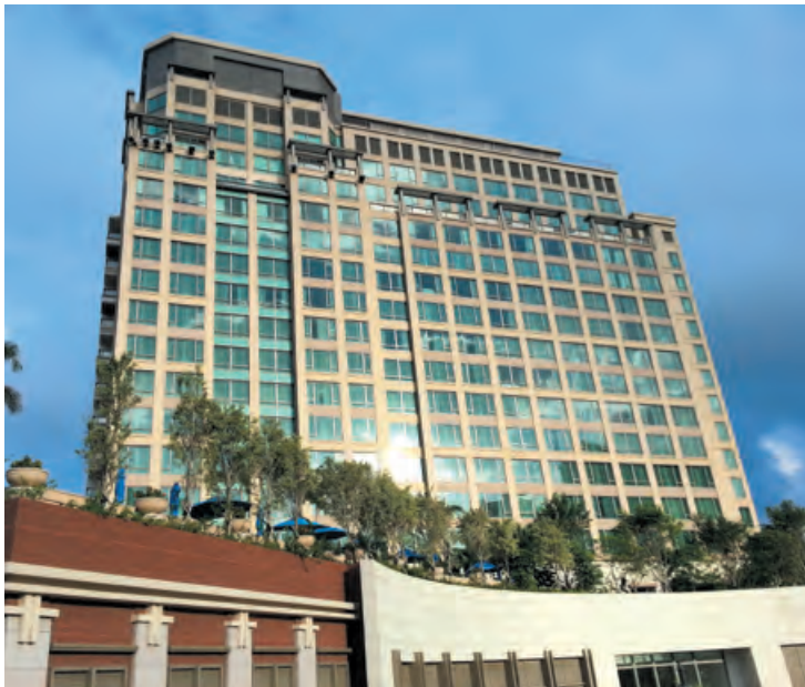
Exterior of the conference and resort hotel at North Area, N3, Discovery Bay, Lantau Island 大嶼山愉景灣北N3區會議及度假酒店的外觀
