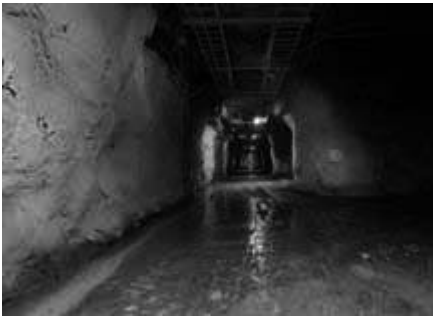
Underground Mining Tunnels
