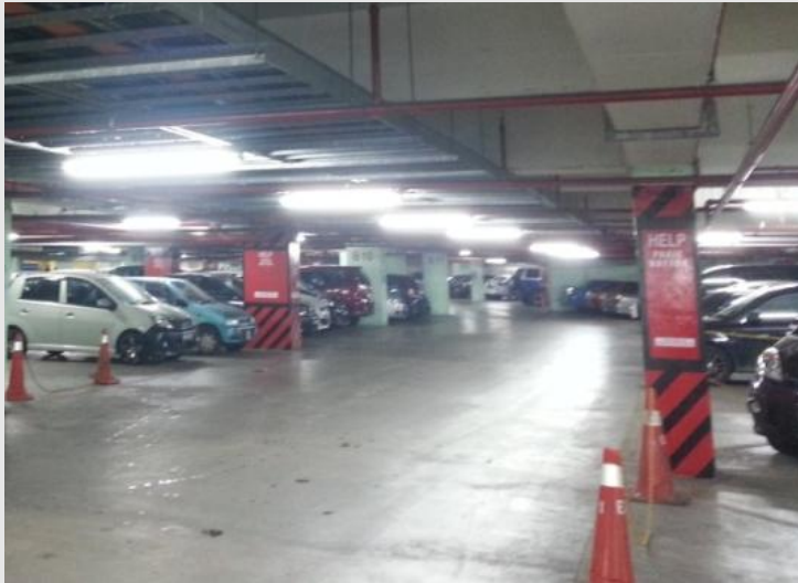
New T5 Lighting at Basement Car Park
