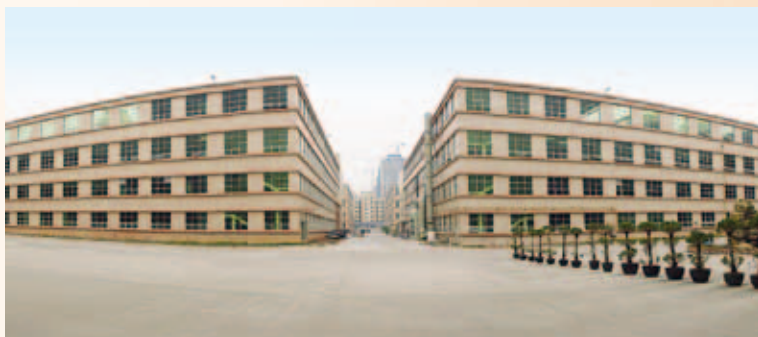
The construction work of the third phase of Daya Bay Industrial Complex (Block 7 & 8) (Left) had been completed 大亞灣工業園第三期(第7、8棟廠房)(圖左)之建築工程已經完成
