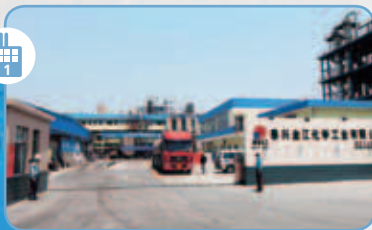
位於江蘇泰興的溶劑廠房 The solvents plant in Taixing, Jiangsu
