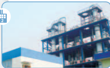
位於廣東江門的溶劑廠房 The solvents plant in Jiangmen, Guangdong
