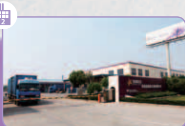
位於上海青浦的塗料廠房 The coatings plant in Qingpu, Shanghai
