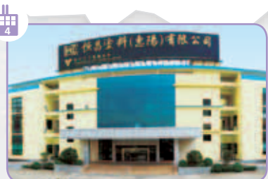
位於廣東惠州的塗料廠房 The coatings plant in Huizhou, Guangdong
