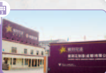
位於四川成都的塗料廠房 The coatings plant in Chengdu, Sichuan
