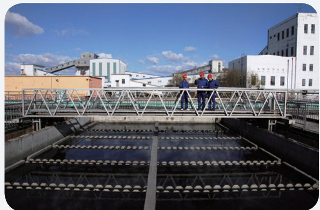
Waste water treatment project
