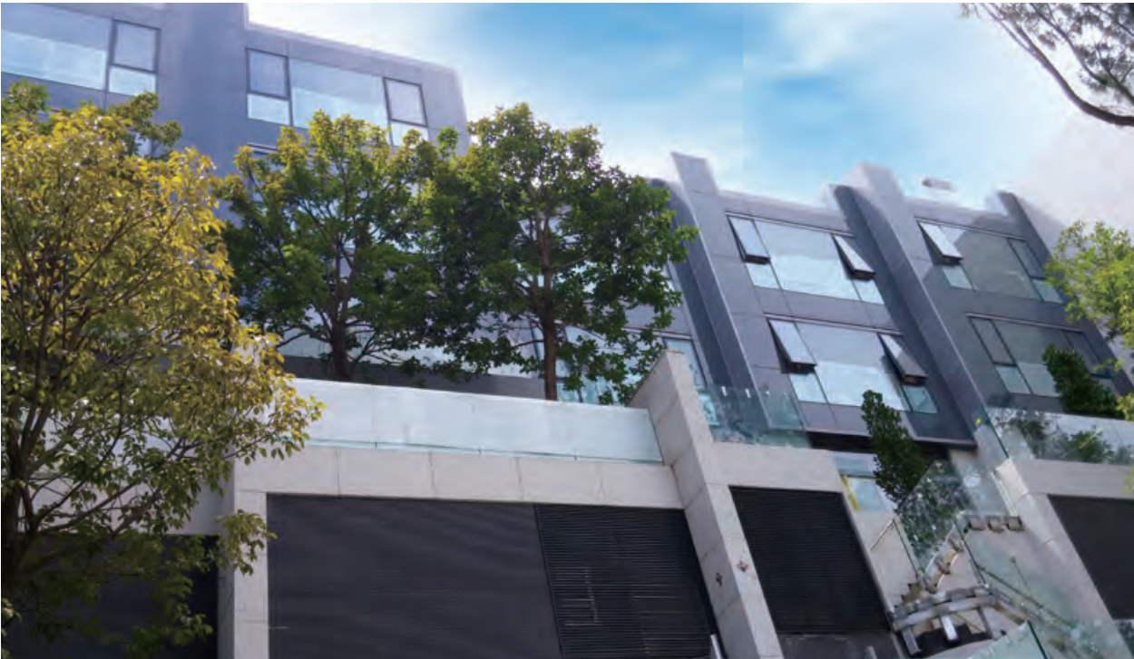
Proposed residential development at No. 62 Begonia Road, Kowloon Tong – curtain wall and aluminium window 九龍塘海棠路62號建議住宅發展項目－幕牆及鋁窗
