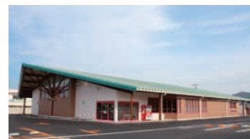
Standardized hall (exterior)
