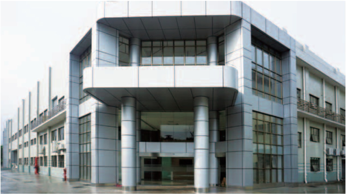
Newly completed manufacturing buildings of WKK Technology Park at Dongguan, China 新完成之中國東莞王氏港建科技城廠房
