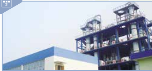
位於廣東江門的溶劑廠房 The solvents plant in Jiangmen, Guangdong
