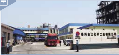
位於江蘇泰興的溶劑廠房 The solvents plant in Taixing, Jiangsu
