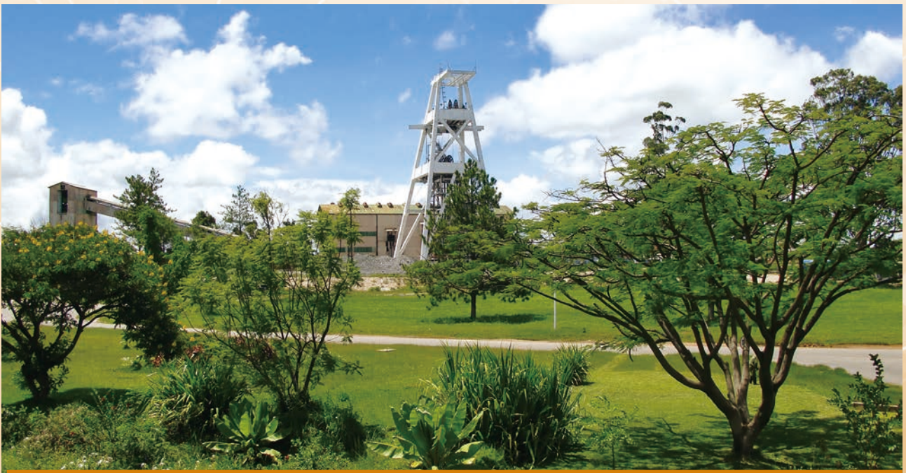
Chambishi銅礦主井架
