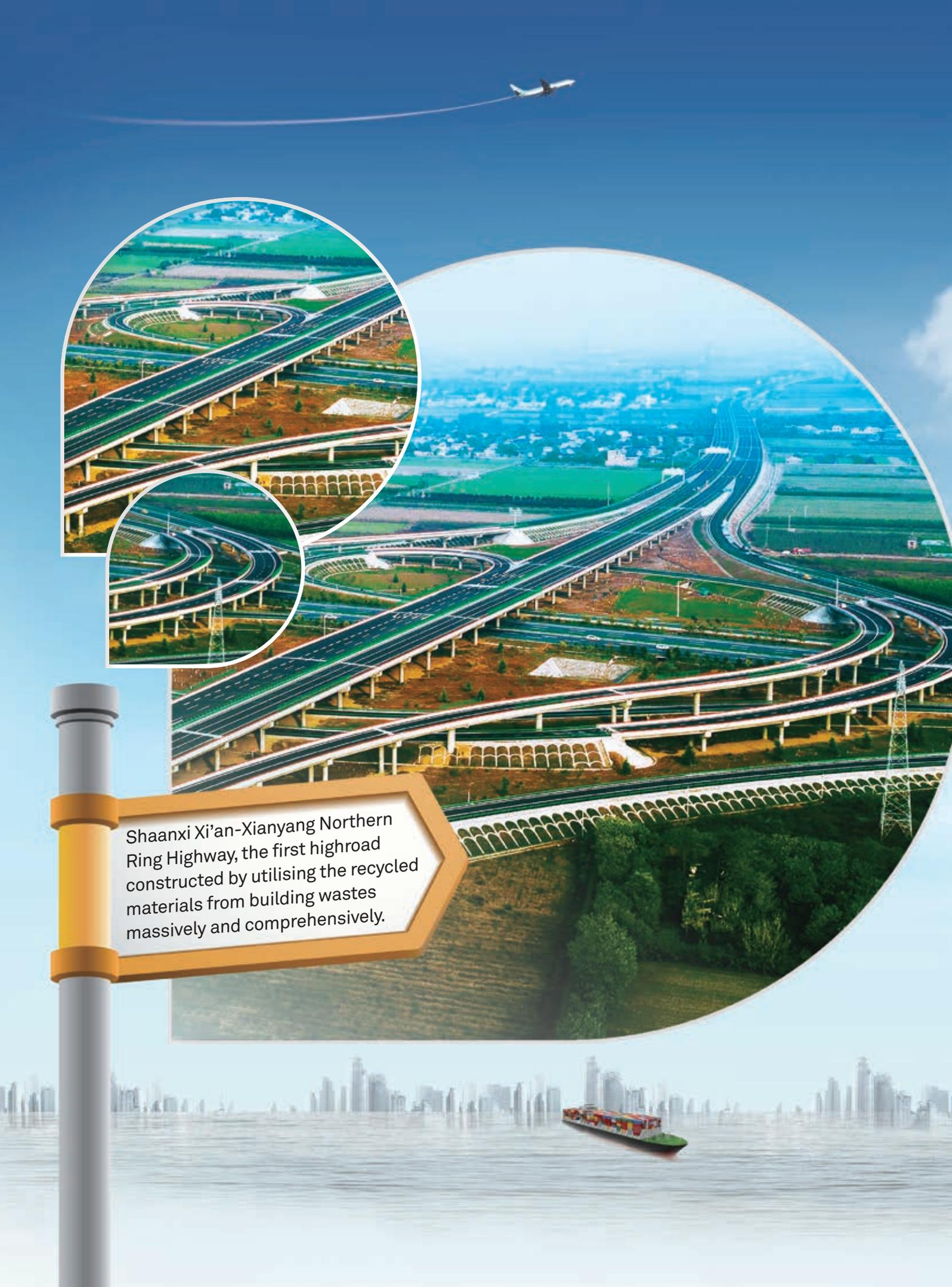
Shaanxi Xi'an-Xianyang Northern Ring Highway, the first highroad constructed by utilising the recycled materials from building wastes massively and comprehensively.
