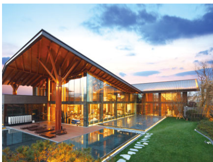
蘇州北辰旭輝壹號院 Suzhou North Star CIFI No.1 Courtyard
