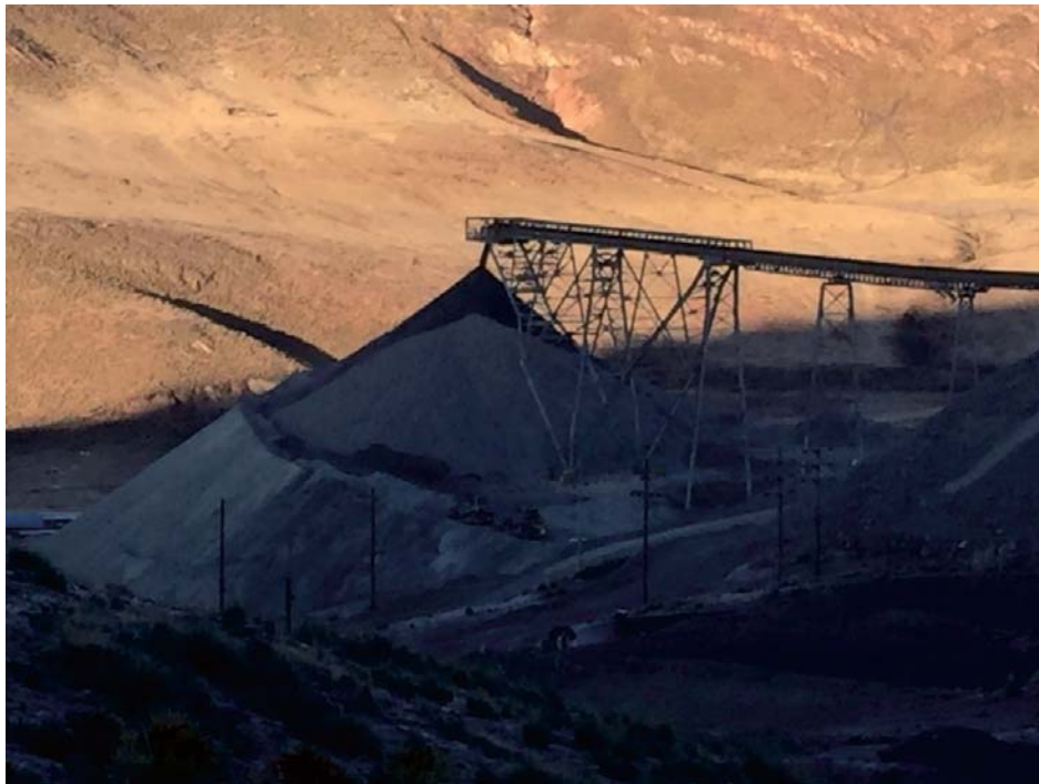
Figure 61: Crushed ore stockpile – July 2016
