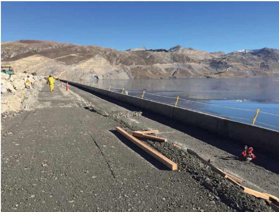
Figure 72: Tailings dam wall construction – July 2016
