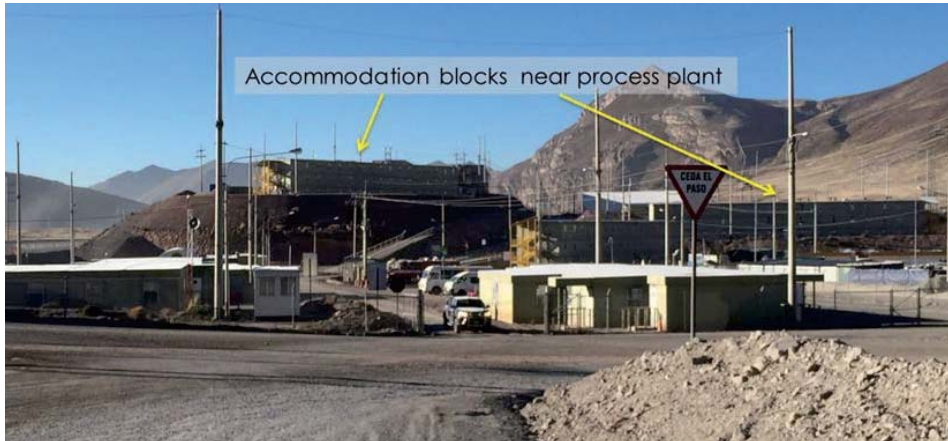
Figure 74: Accommodation blocks and camp adjacent to process plant facility 2016-July-27
