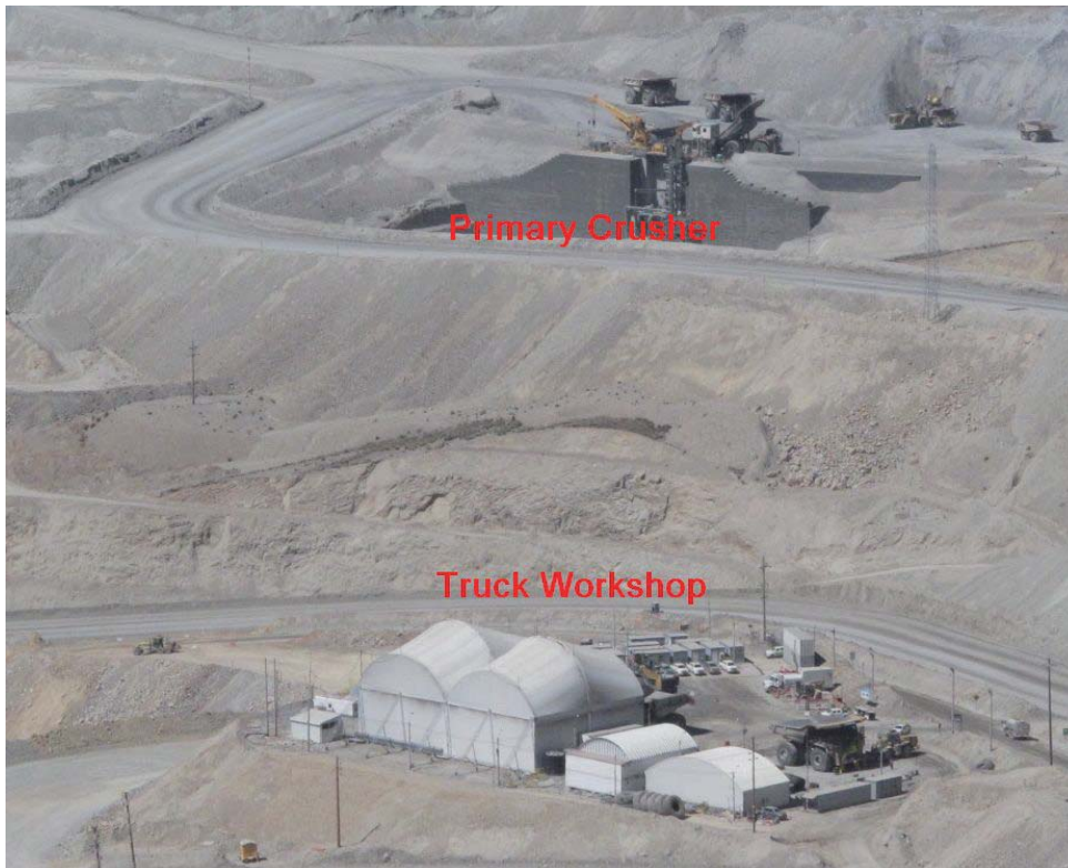
Figure 64: Truck workshop and light vehicle workshop facilities – July 2016
