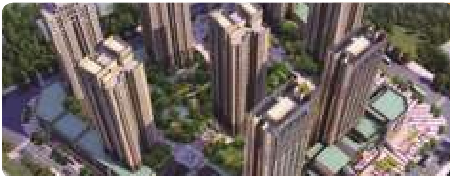
Chongqing Panlong Jinmao Residence
