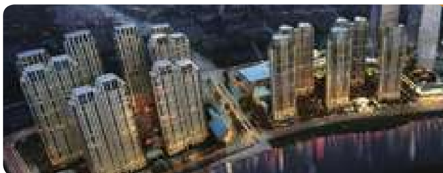
Changsha Meixi Lake Jinmao Palace situated inside Changsha Meixi Lake Jinmao Plaza
