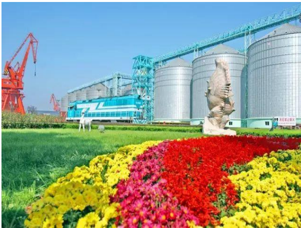
大港港區糧食儲罐
