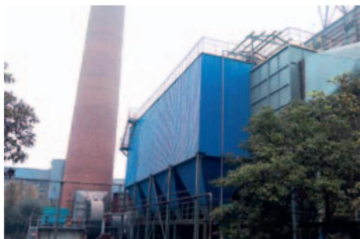
1#Sintering machine tail dust removal efficiency enhancement
