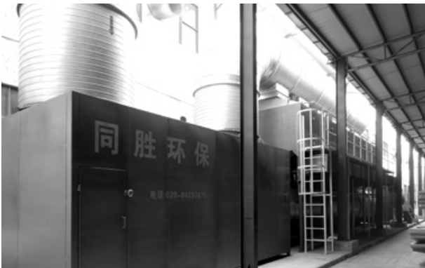
Organic air emission treatment facilities 有機廢氣處理設備
