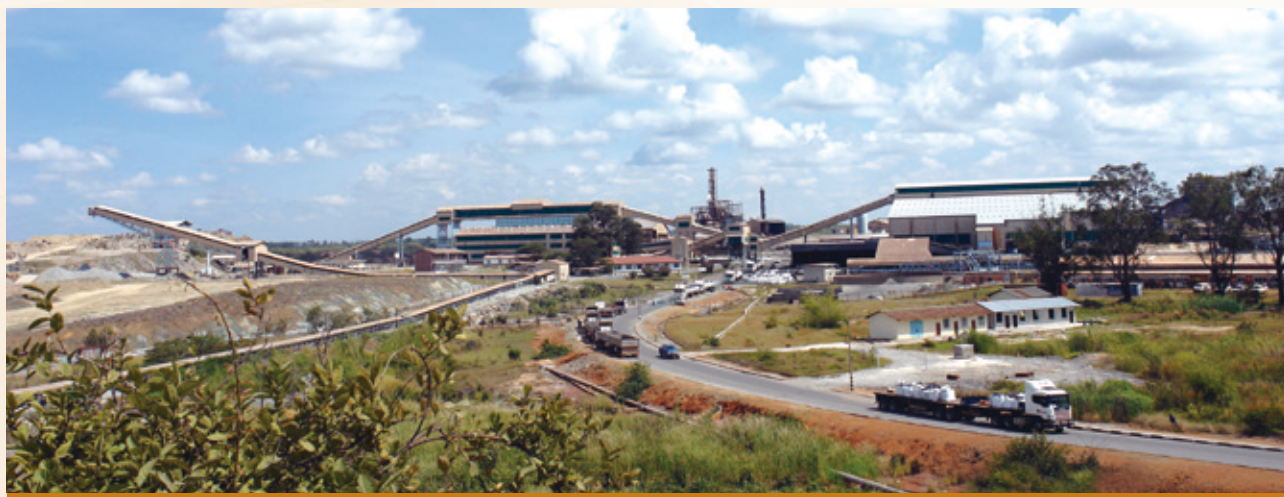
Chambishi銅礦選礦廠全景
