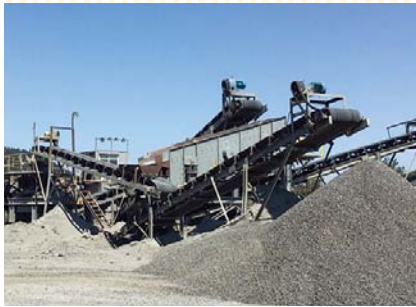
Crusher installed in Plot H H區裝置之碎石機
